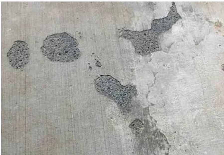
Fig 3: Concrete Blisters
