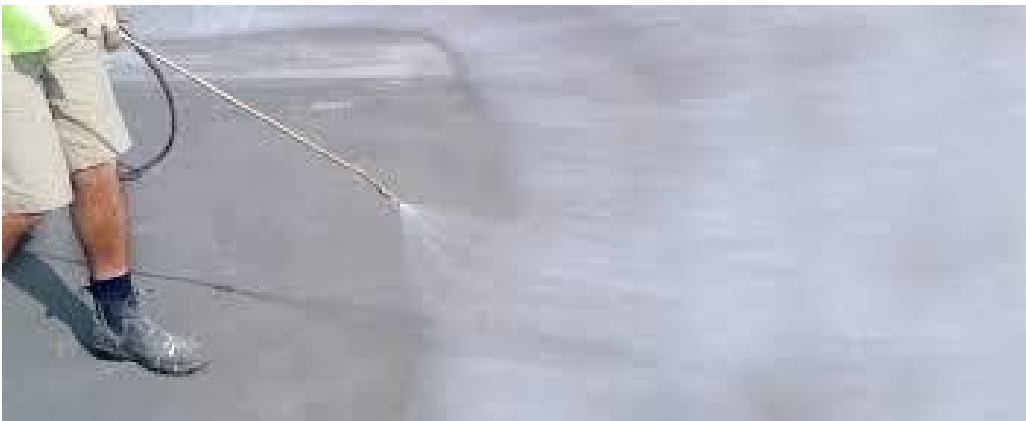
Fig.: Curing by the sprinkling of water
