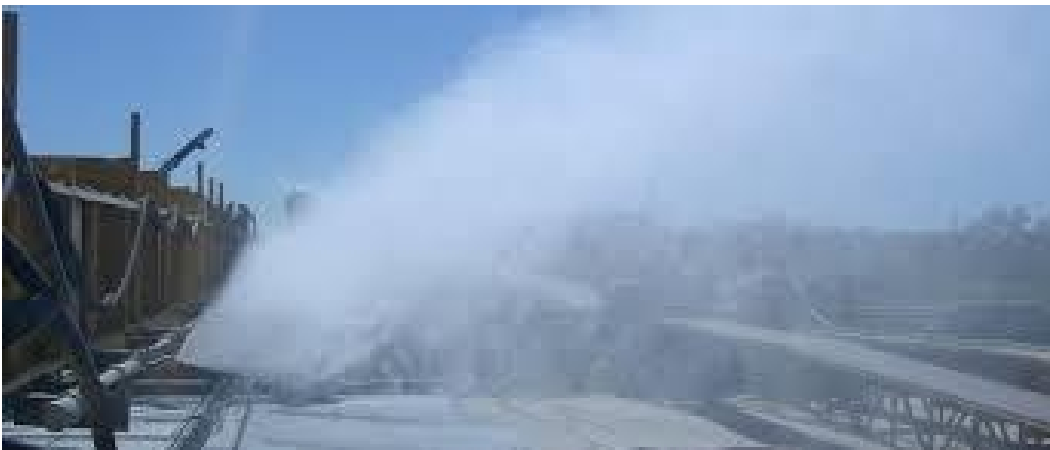
Fig.: Steam curing of concrete
