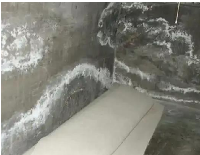
Fig 7: Efflorescence
