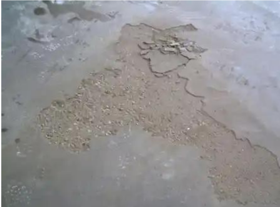
Fig 4: Delamination
