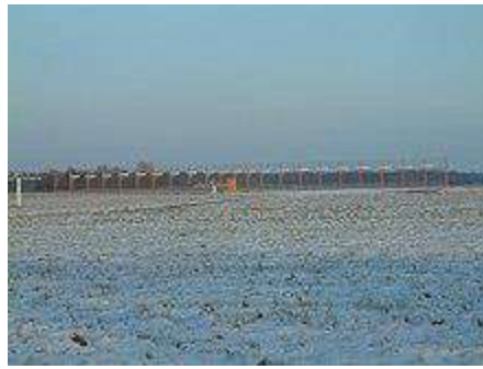
The localizer station for runway
